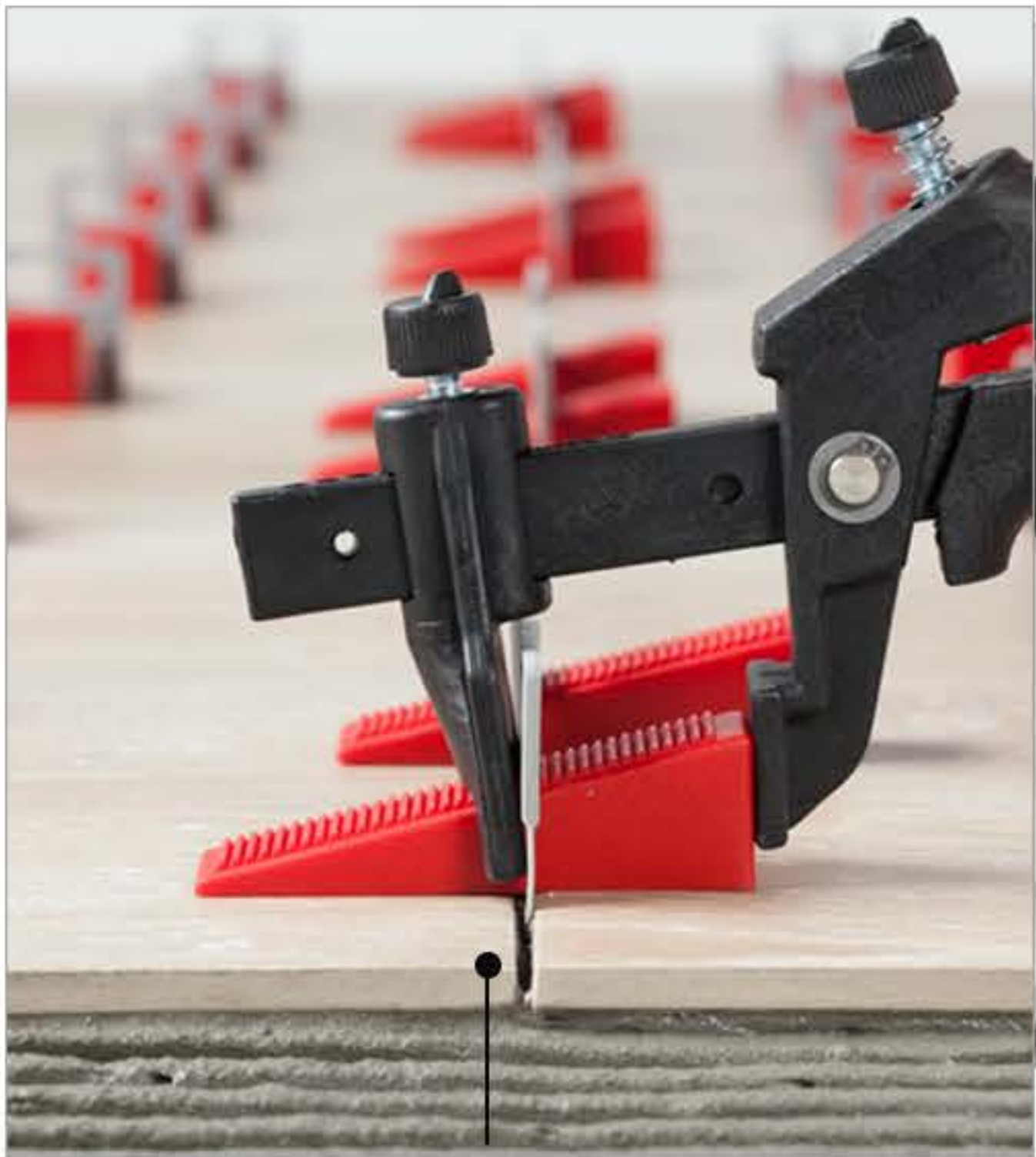
Using the precision application tool allows accurate levelling of the tile.
